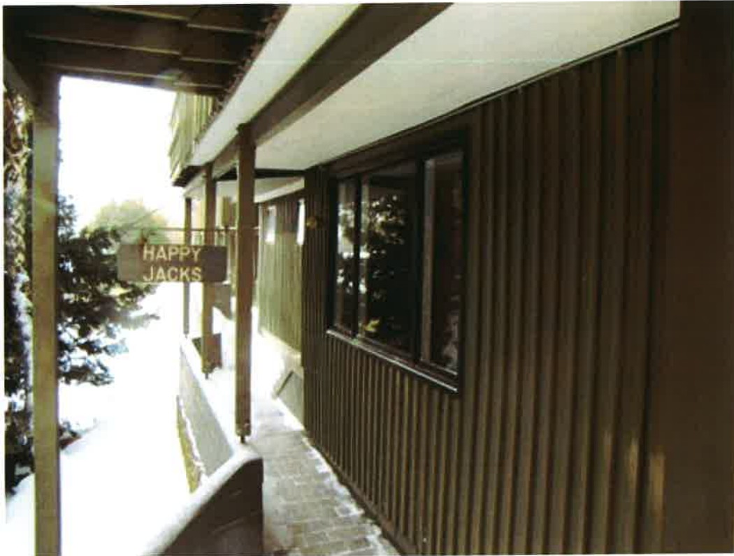
Figure 2: Undercroft of balcony over, looking towards Unit 9 entry
